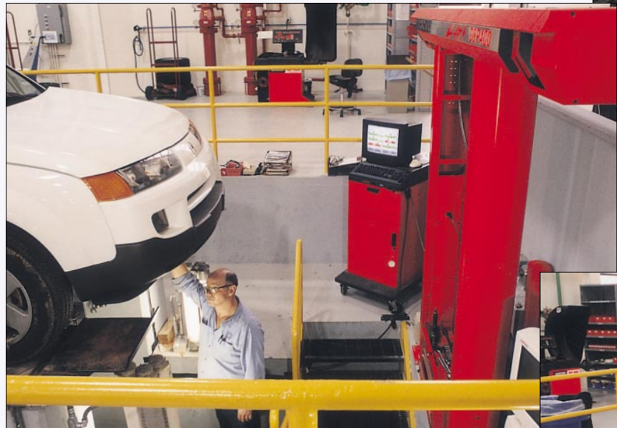
Mirroring a typical shop configuration, the Hunter-equipped test bays include an upper and lower pit for quick and convenient access to a vehicle's wheel wells and underside.
