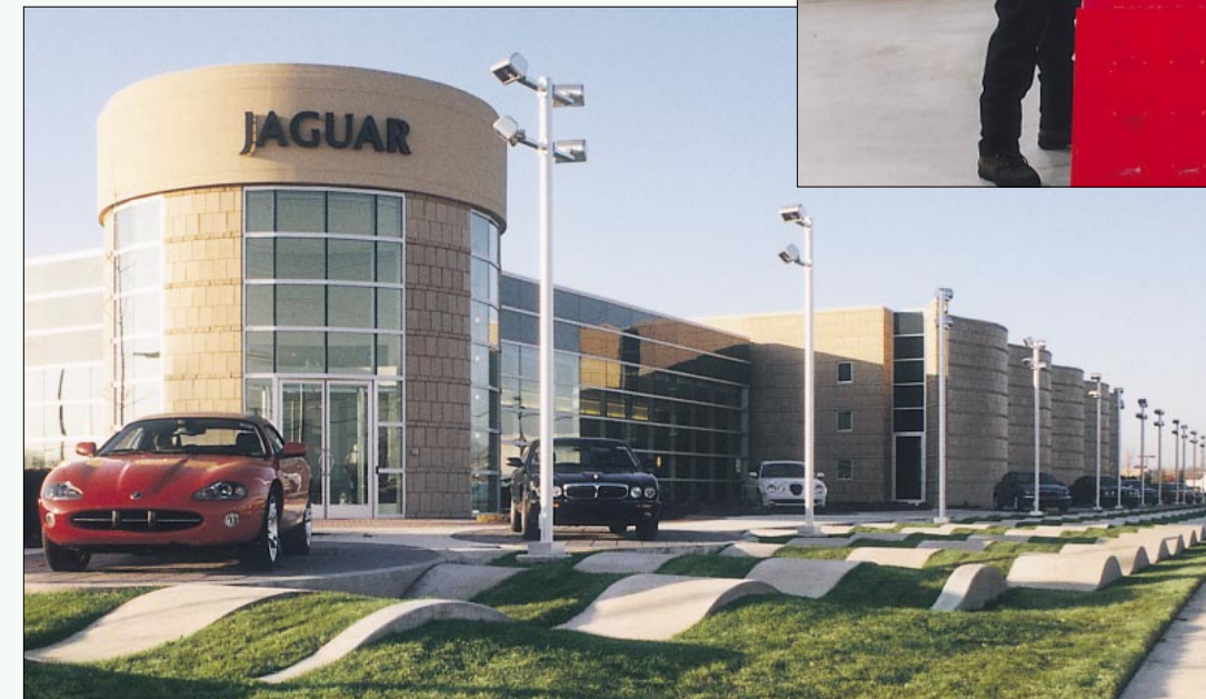
Jaguar of Novi's sophisticated building design is a testament to the luxury and quality embodied in the cars sold and serviced at the Michigan dealership. The 38,000 square foot facility includes a service department that is almost exclusively Hunter-equipped.
